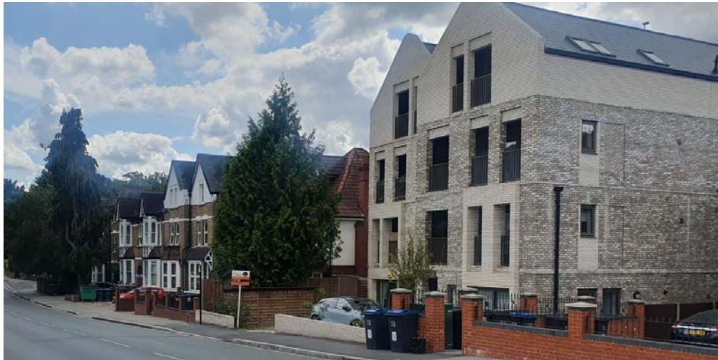
Figure 5: Picture taken from St Peter's Road illustrating roof forms
